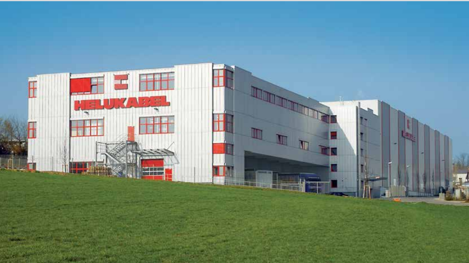
HELUKABEL® Headquarters Hemmingen/Stuttgart, Germany
